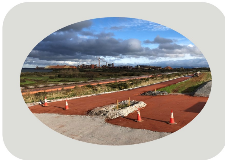
Figure 4. RemovAL sub-base construction and aerial view of finish RemovAL pilot road.
